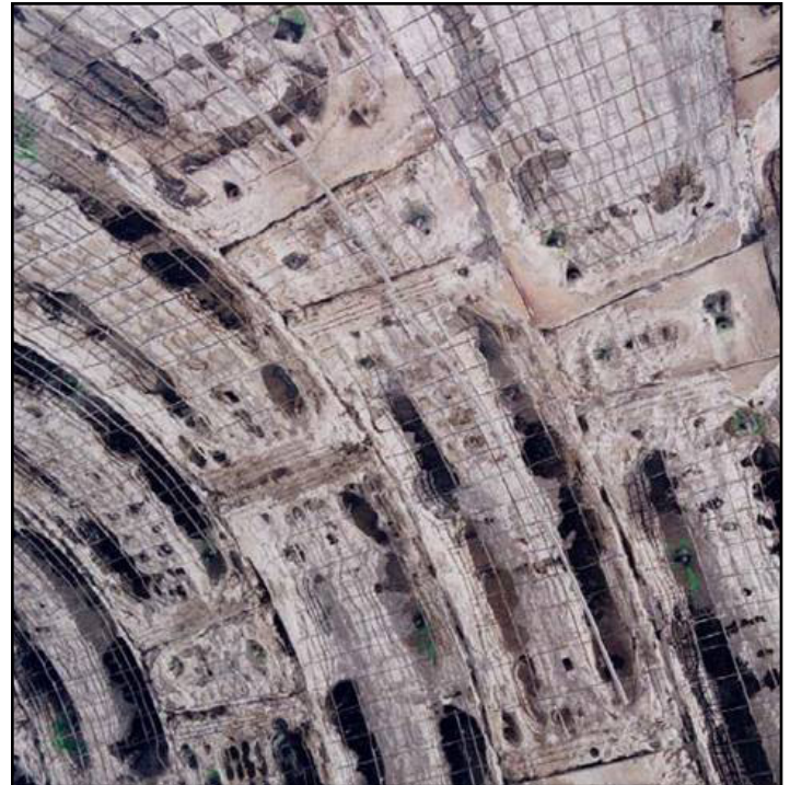
Figure 1: Fire induced spalling damage in the tunnel lining of the Channel Tunnel between England and France.
